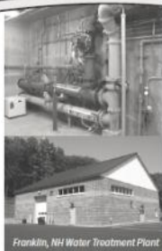
Franklin, NH Water Treatment Plant
