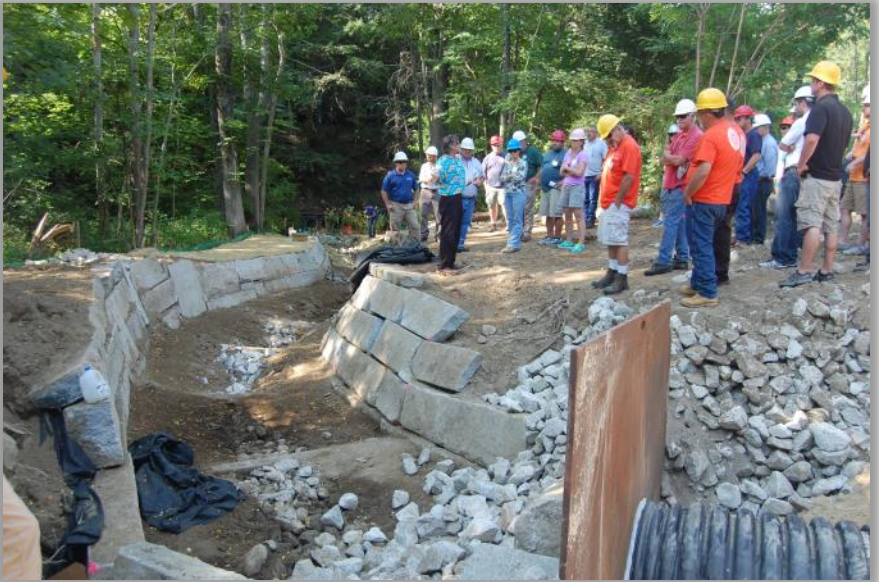
Drainage repair work, Dover, NH.
