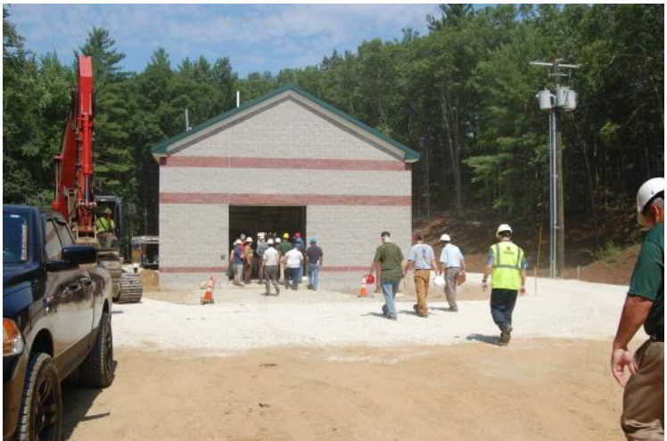
Dover's new chemical feed facility for the Calderwood and Campbell Wells.
