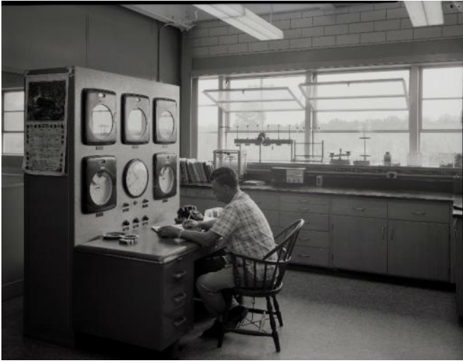
Portsmouth's water system controls in 1968.
