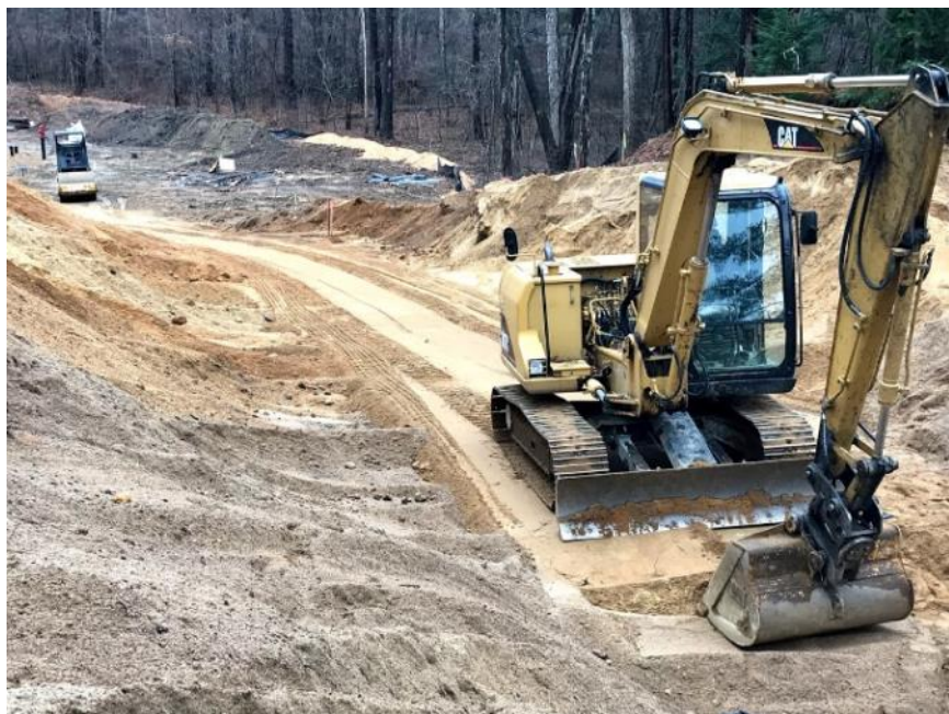
Figure 3 - Well 4 & 5 Access Road
