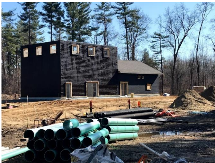
Figure 4 - Well 4 & 5 WTP Structure
