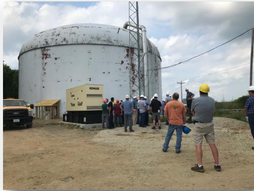
The Newington Tank, a 1.5 MG tank constructed in 1957 at the site of the Newington Booster Pump Station—Construction Field Day 2019.
