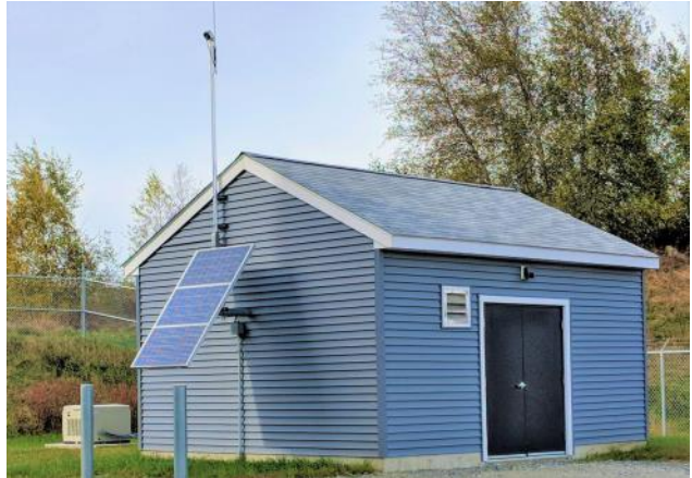
Utility building with solar panel and standby LPG Genset
