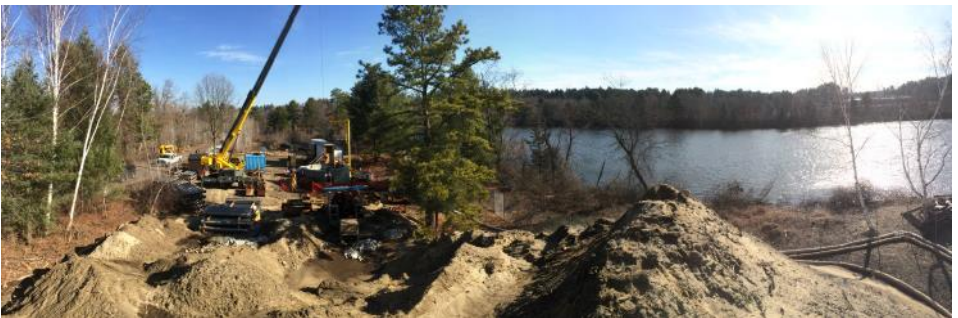
Radial well construction site on the Merrimack River.
