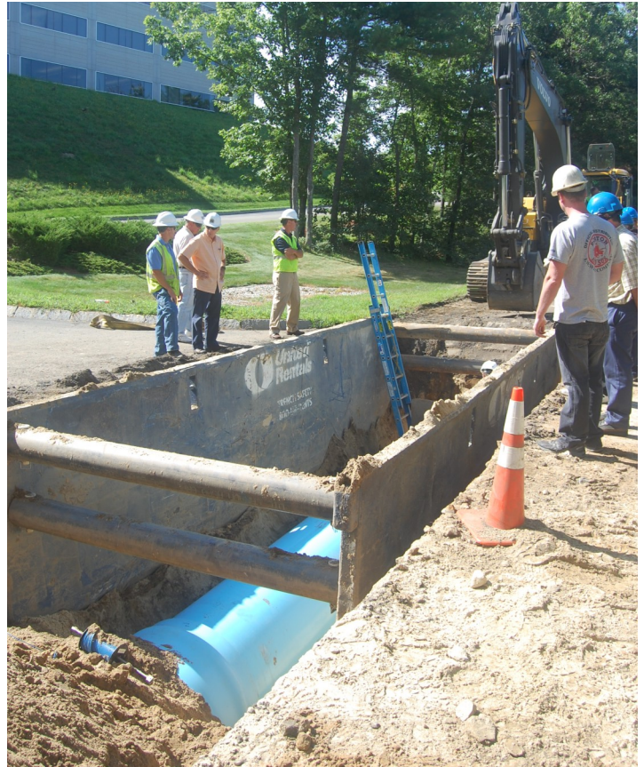
Construction Day 2015—Pennichuck's Merrimack River transmission main.
