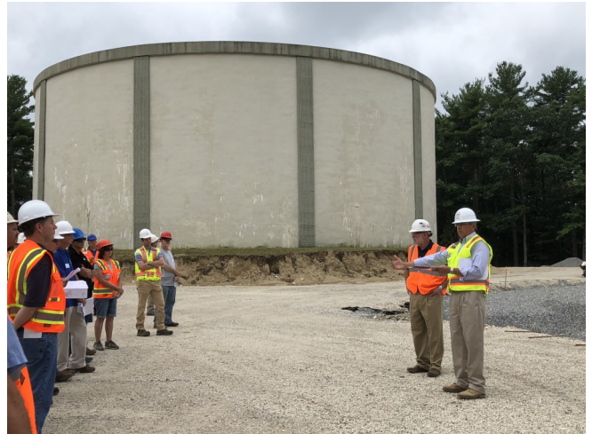
Construction Field Day in August 2018 at the site of a 3MG Manchester Water Works storage tank in Londonderry.
