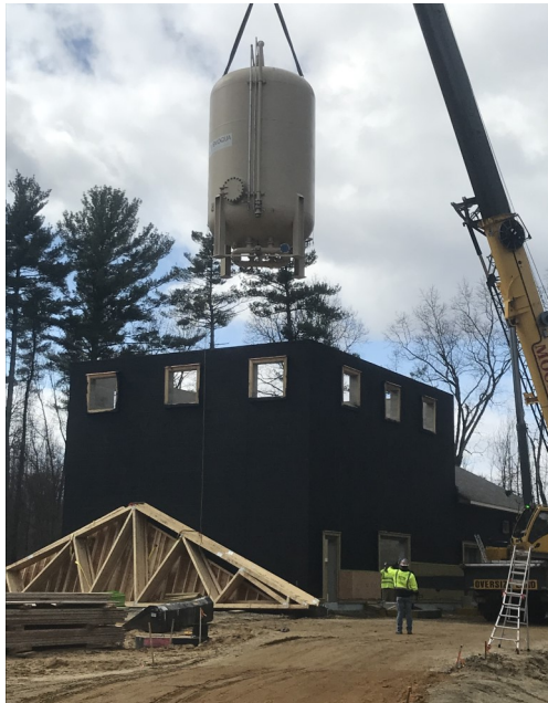
GAC Vessels being set at the Well 4&5 WTP structure.
