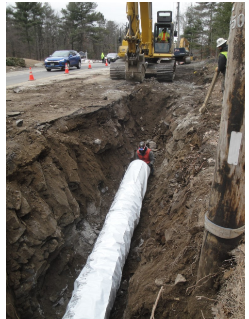
20-inch ductile iron water main installation along Route 28 in
