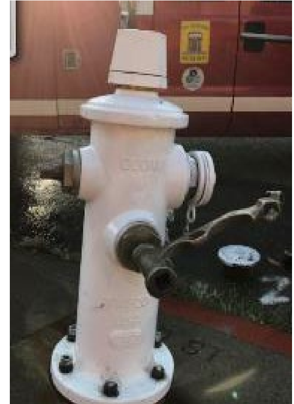
iHYDRANT™ | INSTALLATION, SF
